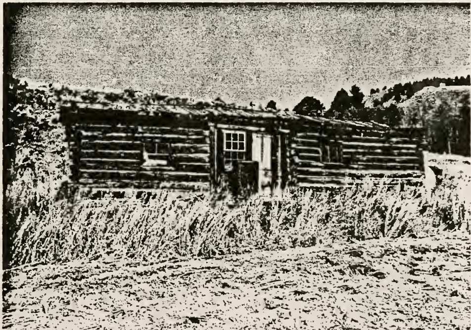
Figure 51. Structure #5, southwest view.
